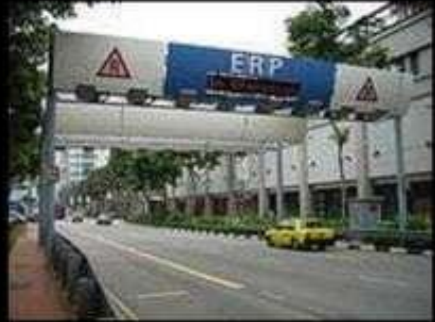
Congestion pricing gantry at North Bridge Road, Singapore.
