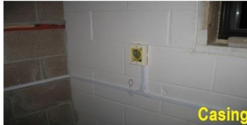
Casing and Capping Electrical Wiring
