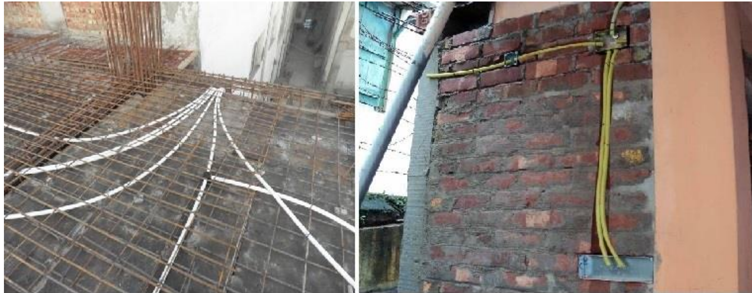
Concealed Conduit Installation in Slabs and Walls
